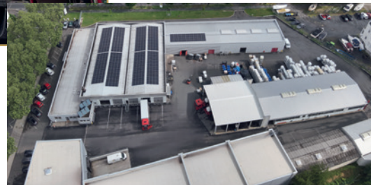
The Wiesbaden site with its new warehouse and photovoltaic system – a commitment to efficiency and sustainability
